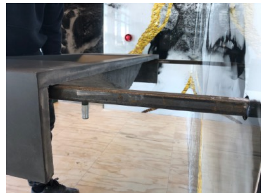
Deposit the vanity on the bracket
