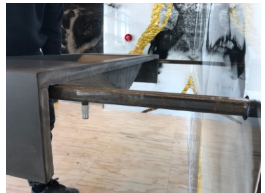
Deposit the vanity on the bracket
