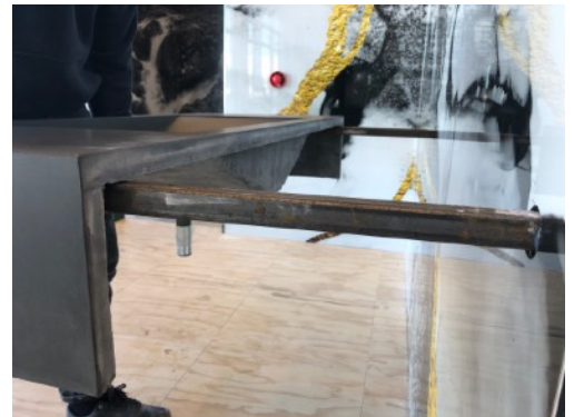
Deposit the vanity on the bracket
