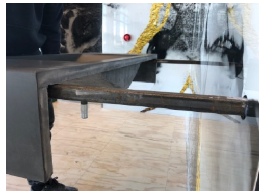
Deposit the vanity on the bracket
