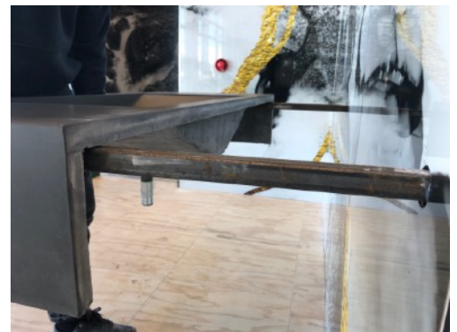
Deposit the vanity on the bracket
